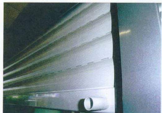
Insulated aluminium-Shutter with ventilation slits.
