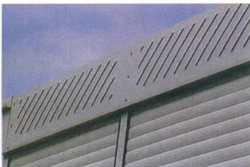
gill-plates for the optimal exchange of air
